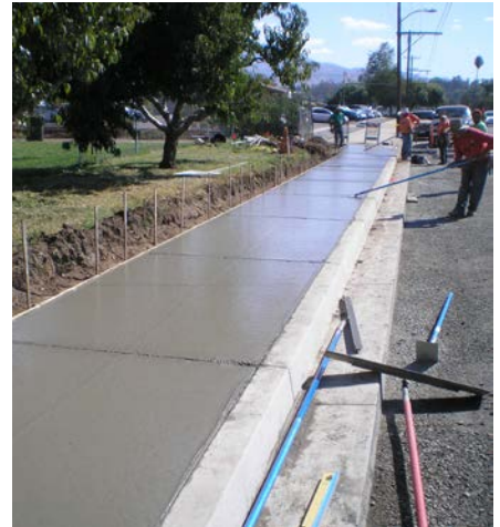
Sidewalk repairs improve the safety and livability of neighborhoods.
