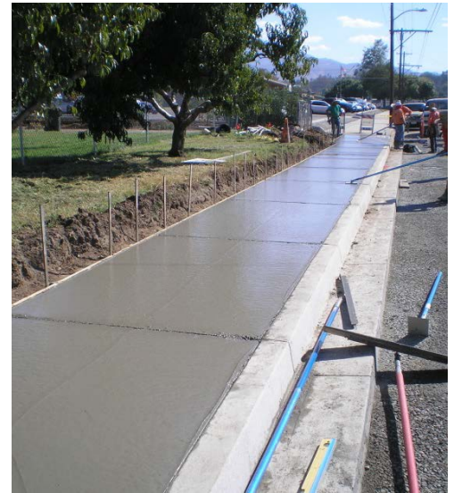
Yucaipa's program to install sidewalks has improved safety in many neighborhoods.
