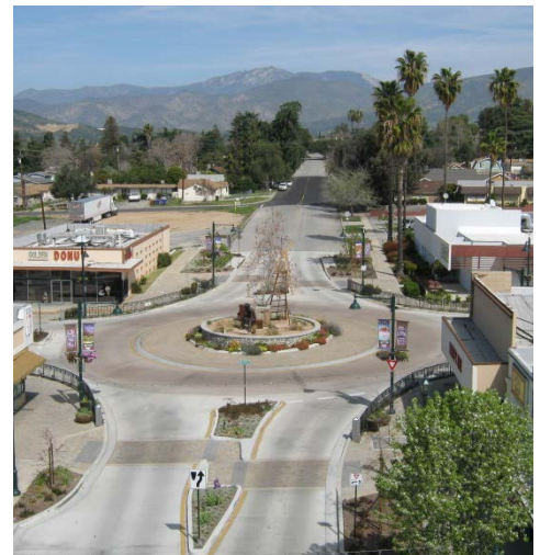
Yucaipa's roundabouts help to calm traffic and create a pedestrian environment in the historic Uptown District.
